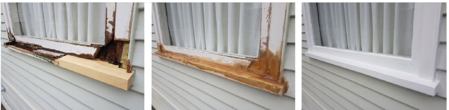
Window Repairs, Australia
